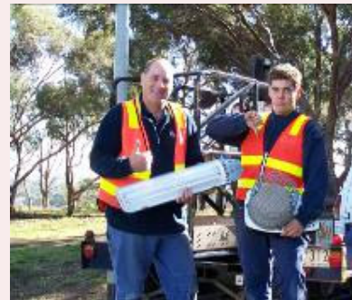
T5 good, MV bad ... Hume Council's electrical contractors replace public lighting.
